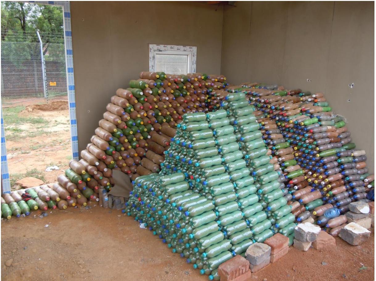
Photograph 2: Photograph of the bottles used to build the wall
