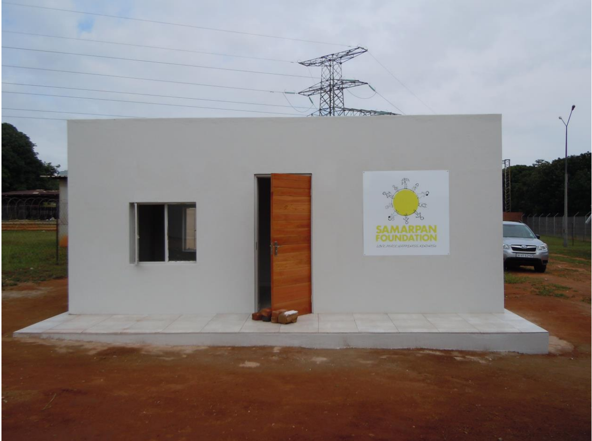
Photograph 1: The building system consists of cold drink bottles that have been filled with sand. The bottles are stacked and the wall covered with a fish net that is then plastered.
