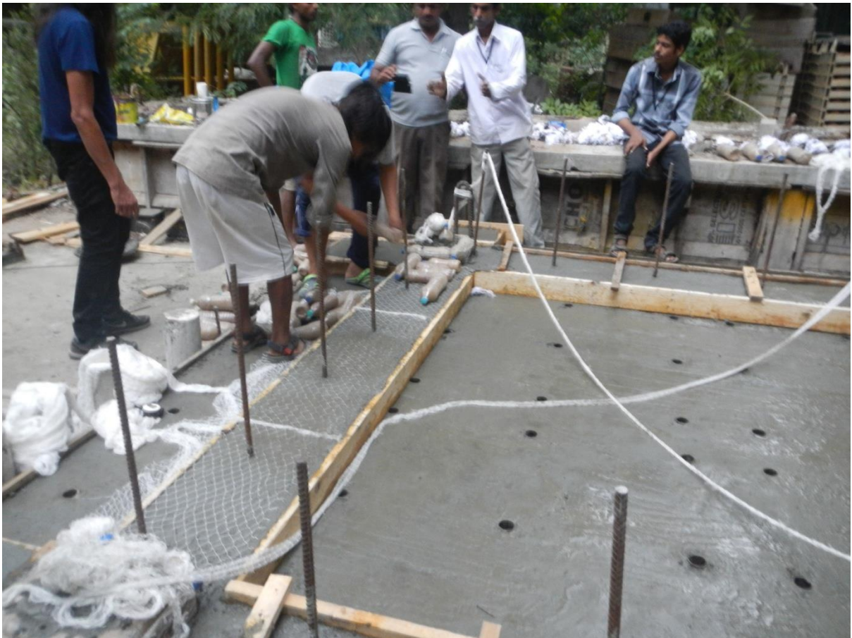
Fig. 6 First layer of PET bottle bricks laid using horizontal staggered bottles on fishnet
