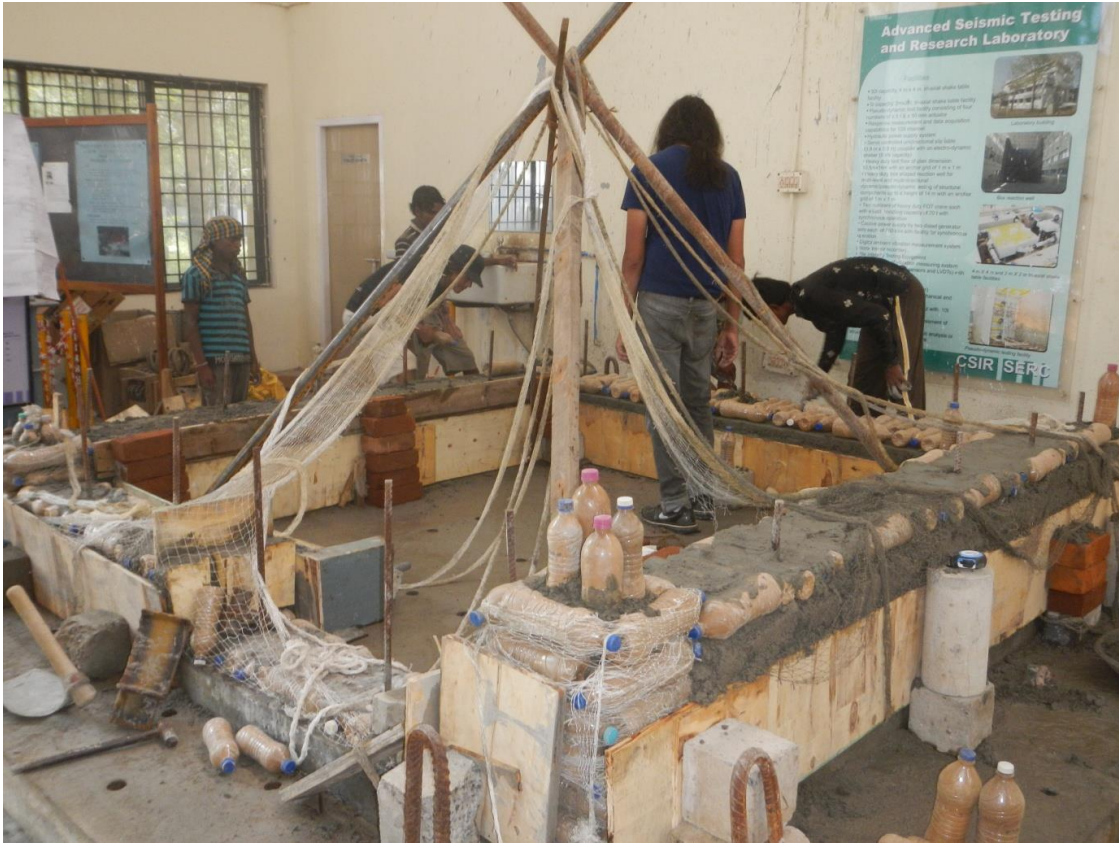
Fig. 9 Construction of PET bottle walls reinforced with Fishnets
