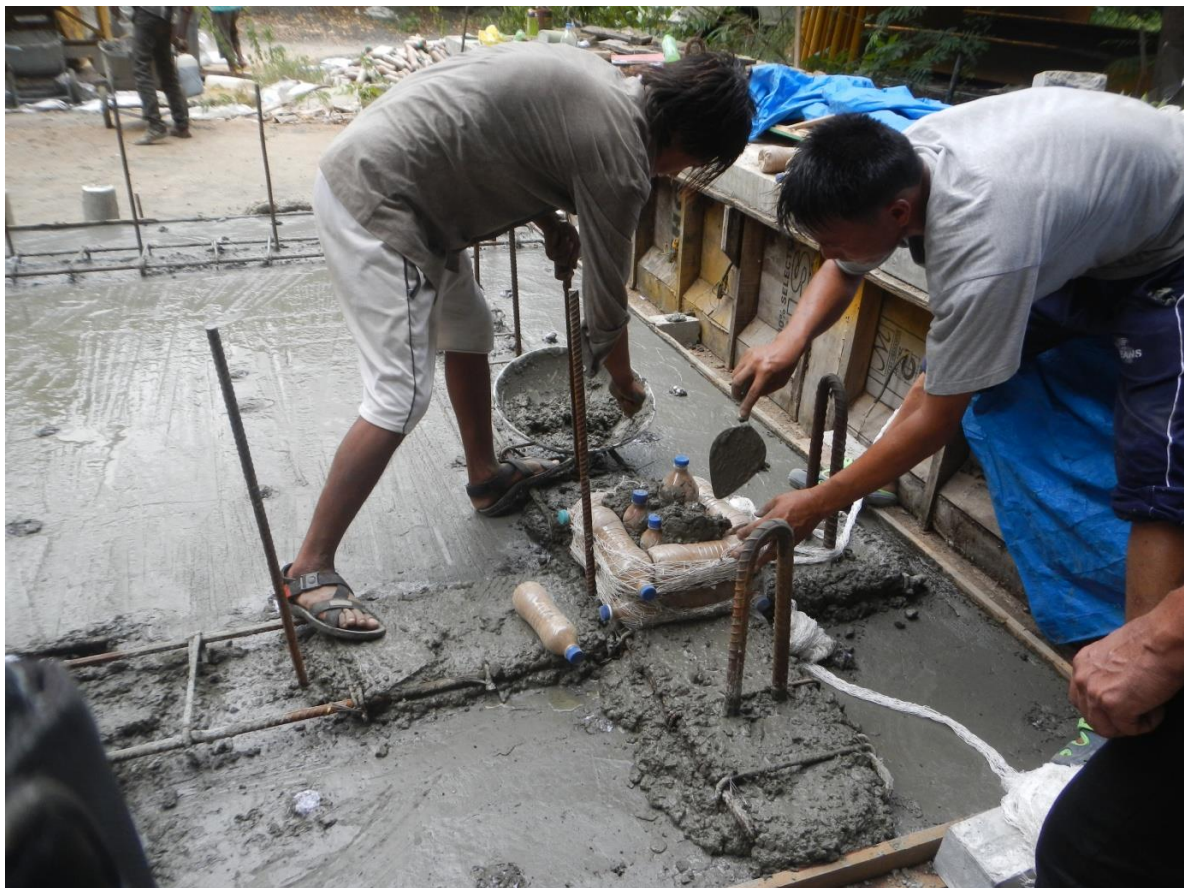
Fig. 4. PET bottle column built using horizontal and vertical bottles wrapped with fishnets
