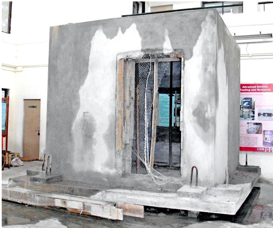
Fig. 16. Finished structure with window and wall opening.
