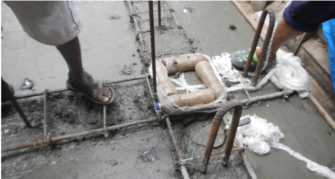
Fig. 3 First layer of PET Bottle Column on fresh concrete slab
