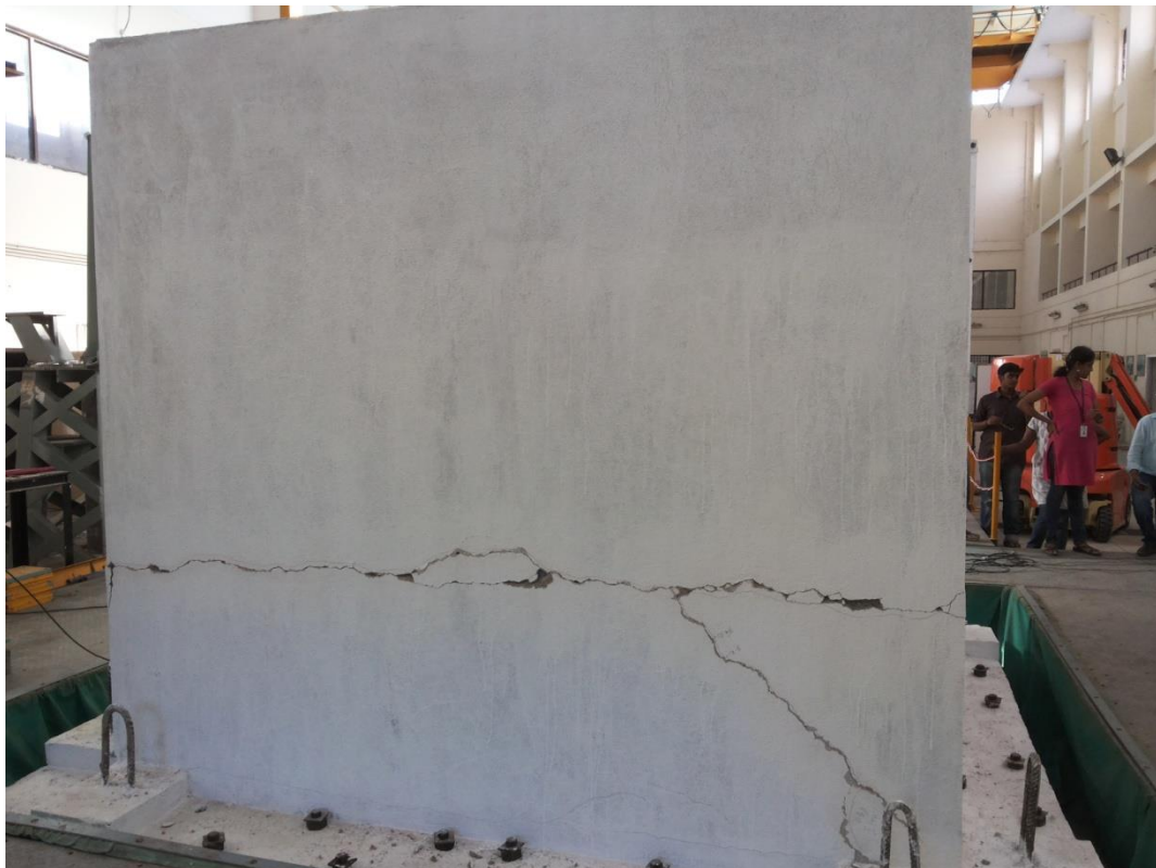
Fig. 33 View of the cracks in the northern solid wall
