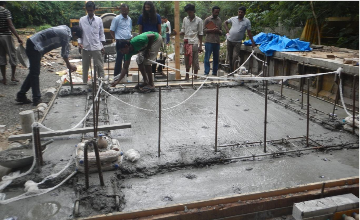
Fig. 5. Overall view of Fishnet arrangement running across to the opposite columns
