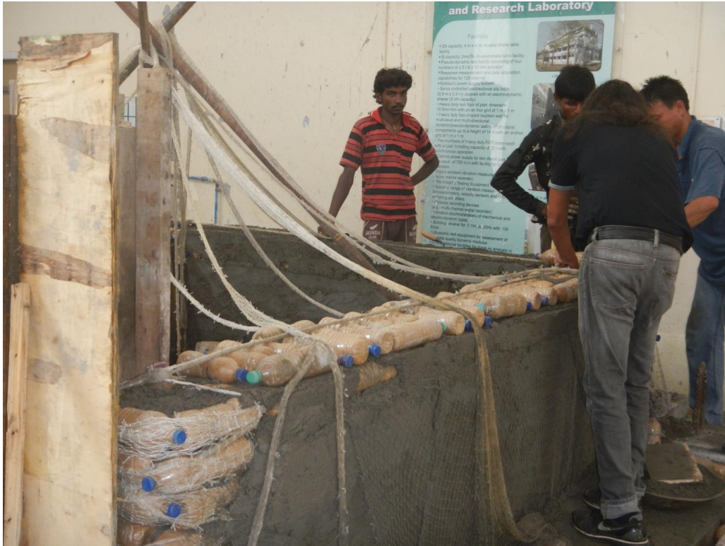
Fig. 11. Construction of PET bottle walls using horizontally staggered PET bottles
