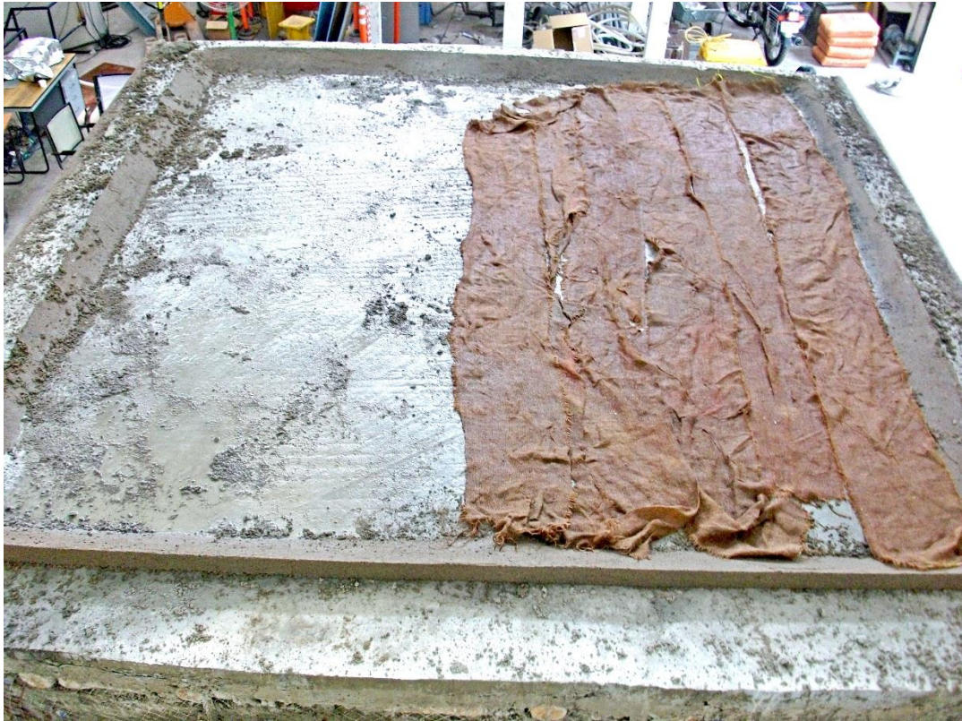
Fig. 15. Finished roof slab under curing.
