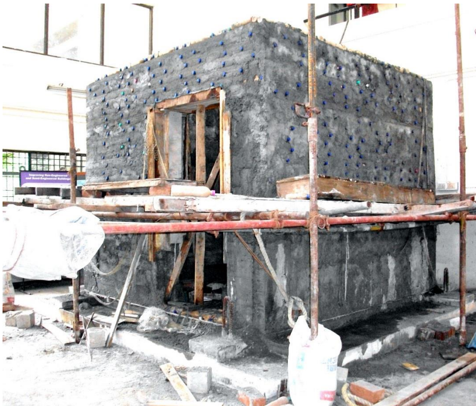
Fig. 12. Completed walls before plastering.
