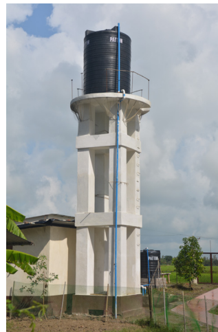
5ft water tower constructed entirely out of PET bottles and fishing net.
